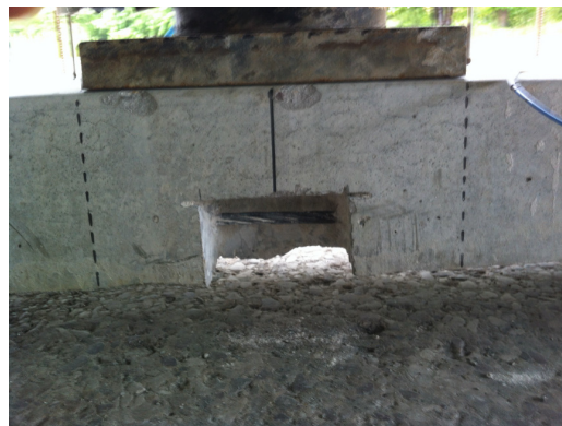
Exposed reinforcement bar to be cut
