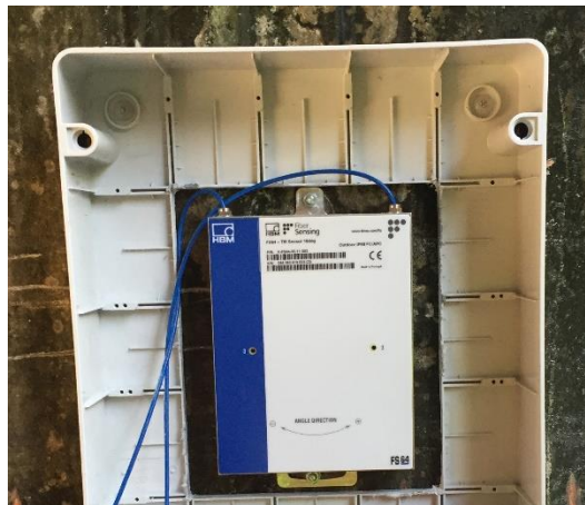
Figure 10: Tilt Meter Installation
