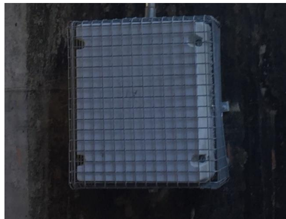
Figure 11: Cage Installation Over Tilt Meters
