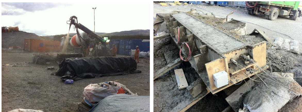
Figure 3: Sprayed Concrete Applied to Beam
